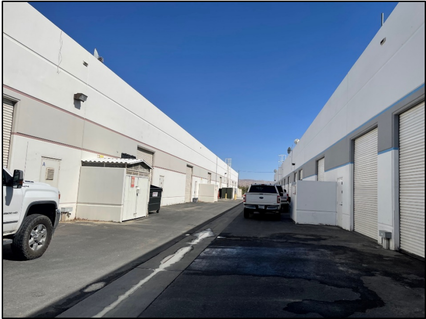
Rear Service Driveway
